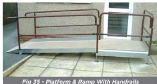
Fig 35 - Platform & Ramp With Handrails
