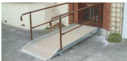
Fig 34 - Self Supporting Ramp With Handrails
