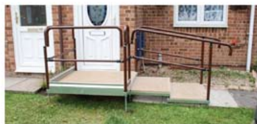
Fig 33 - Platform & Long Tread Steps With Handrails
