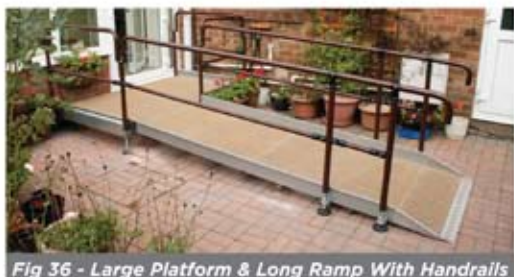
Fig 36 - Large Platform & Long Ramp With Handrails
