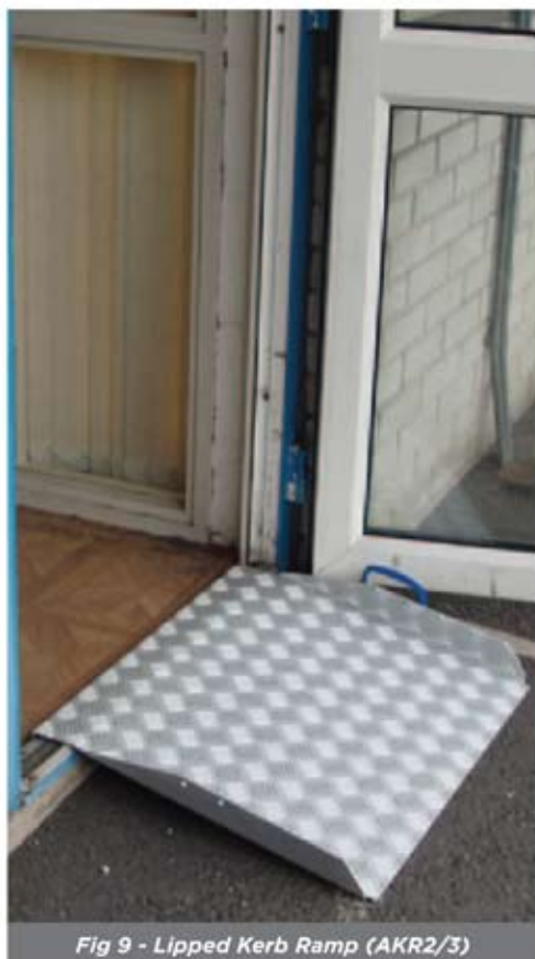
Fig 9 - Lipped Kerb Ramp (AKR2/3)
